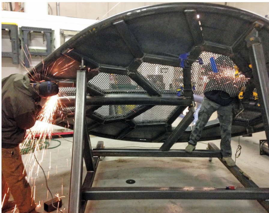
A BSC Custom crewmember welds the steel components of a leaf.
